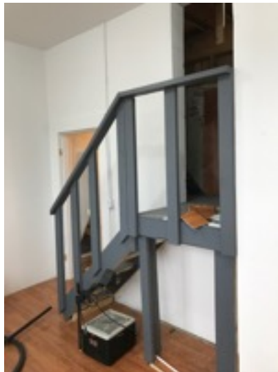
This is a new stair system which allows safe access to the top of the old costume area, the top of the old projection booth, and the catwalk. The picture to the right shows new shelves on top of the old costume room. Work space and storage for our stage lighting equipment will be on top of the old projection booth.
